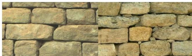
Protection wall at building
