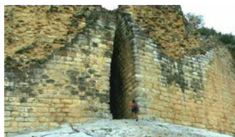
Kuelap – limestone wall
